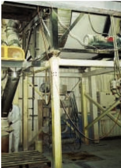
A worker dispenses the coated material from the holding bin and packages it.
